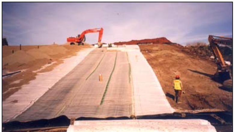
The 4.4 x 100 m rolls of Pozidrain ensured rapid and efficient installation on this large area, including 1 in 4 slopes. Erosamat Type 1A biodegradable erosion control mat was installed to protect slopes.
